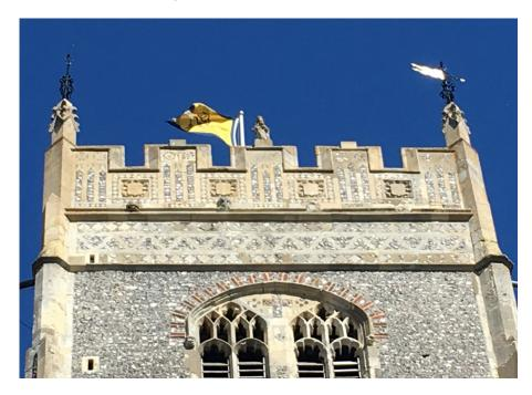
The parapet is an amazing showpiece of flushwork patterns and motifs. It is a double parapet, which is a feature of Suffolk towers, the lower section having a scrolly pattern and the upper embattled part enriched with tracery panels and stone shields set in borders of lozenges. Above, in the battlements, are tiny and exquisite panels, including 'M's, the Aldryche motif and other designs.
