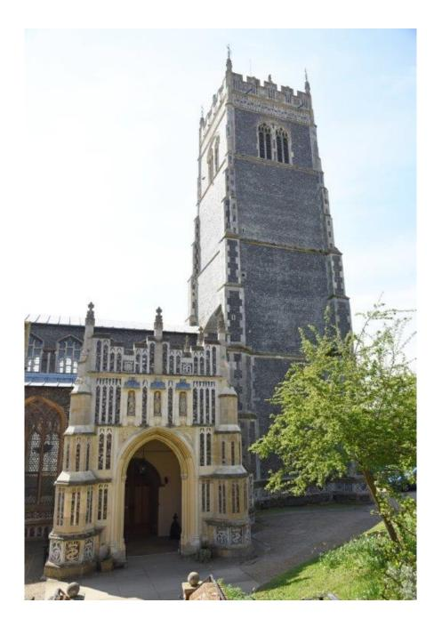
forming a base for the magnificent five-light west window – the largest and grandest in the building. The bell-chamber windows are unusual and elegant. They are pairs of double openings set beneath a hoodmould (to deflect rainwater), but with simple flushwork between, similar to those at Elmswell – another Aldryche tower.
