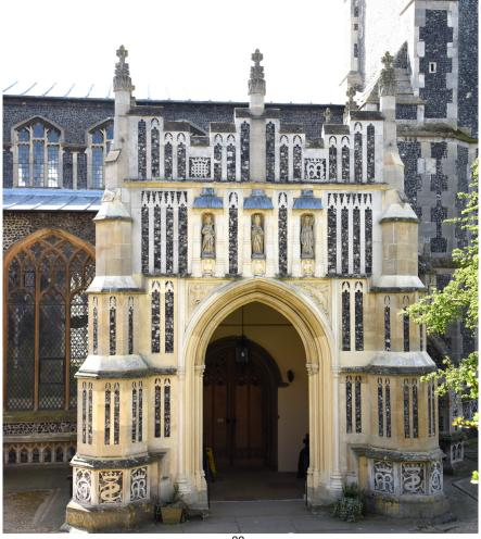
After a very generous donation, in 2017-8 Abbeygate Mason and F A Valiant of Bury St Edmunds renovated the North Porch, by repointing knapped flints, repairing coping stones, niches, leadwork, door, buttresses, the roof and the lime plaster.
